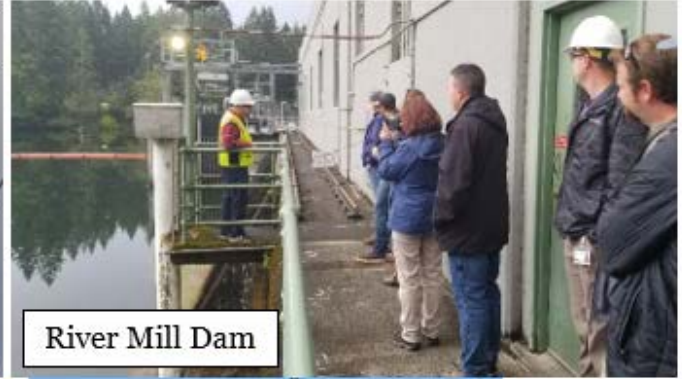
River Mill Dam
