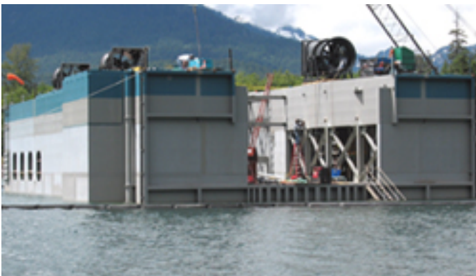
Upper Baker Dam's new "Floating Surface Collector Concrete, WA
