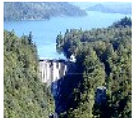
Lower Baker Dam Concrete, WA
